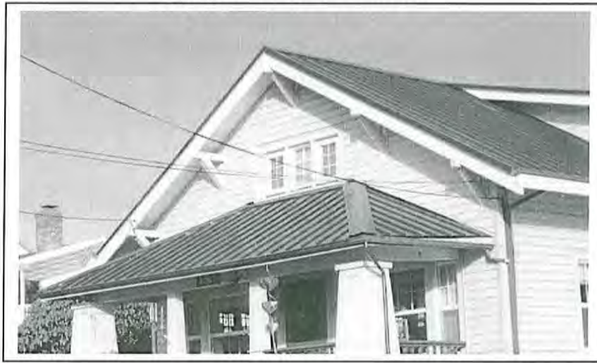
High profile metal seam roof
