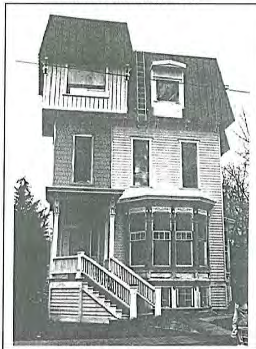
False mansard roof
